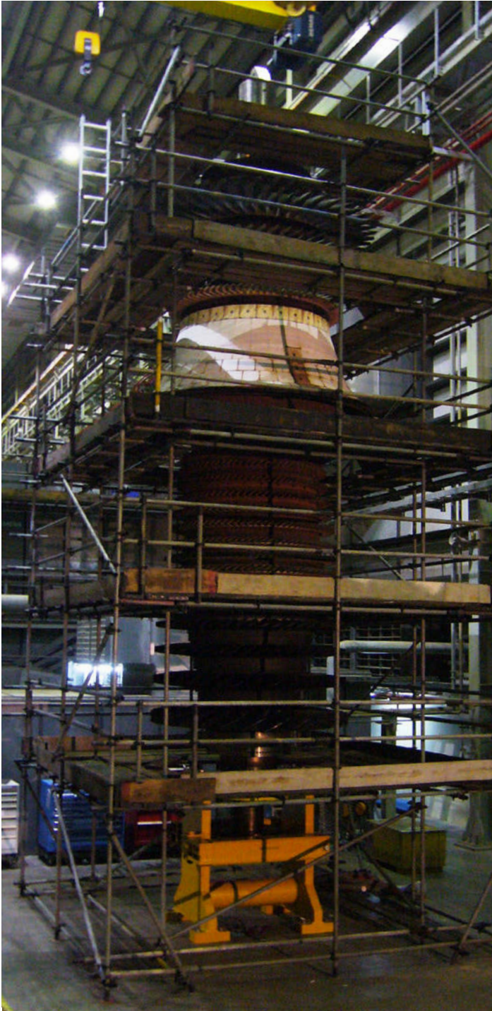
■ BS scaffold tower for GT 94.3 (indoor)
