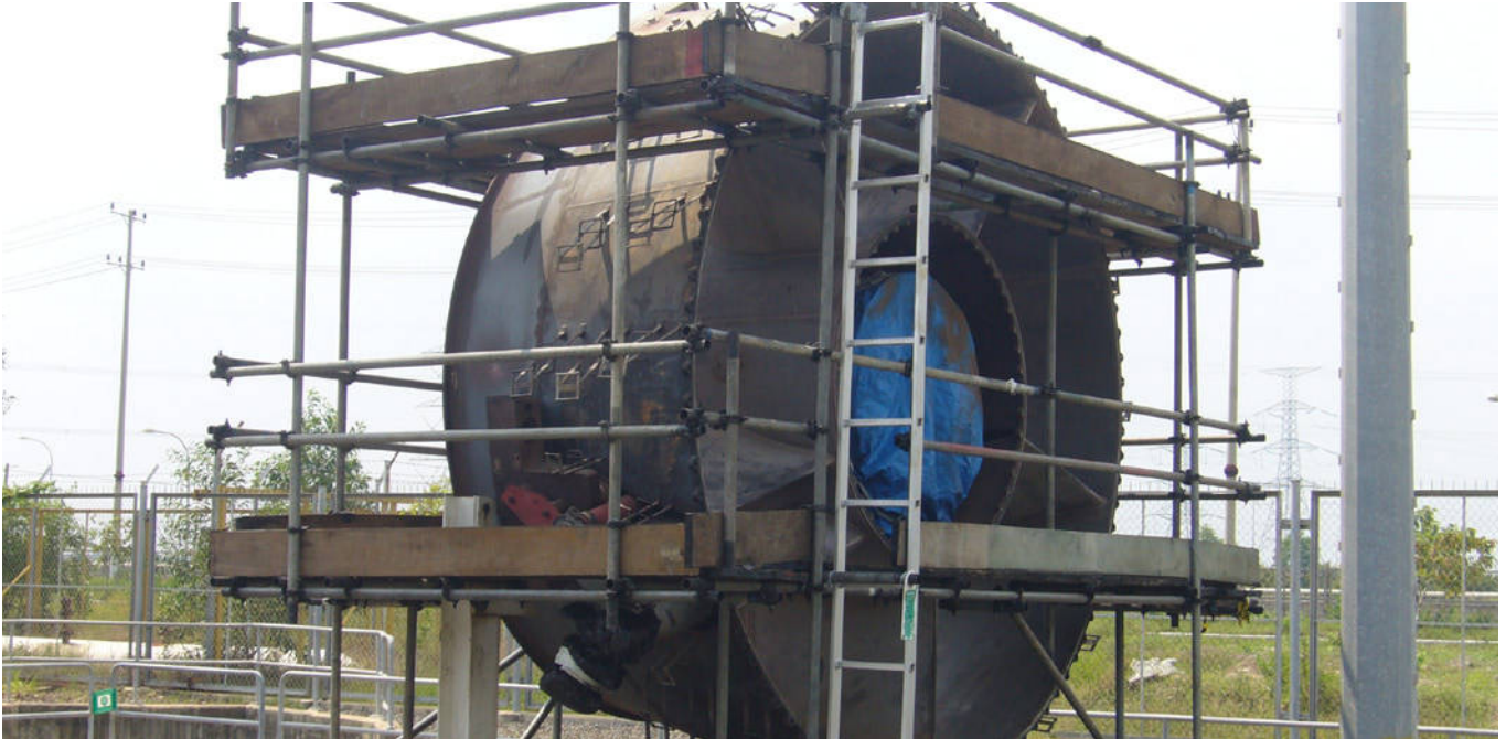
■ BS scaffold tower for GT 94.3 (outdoor)
