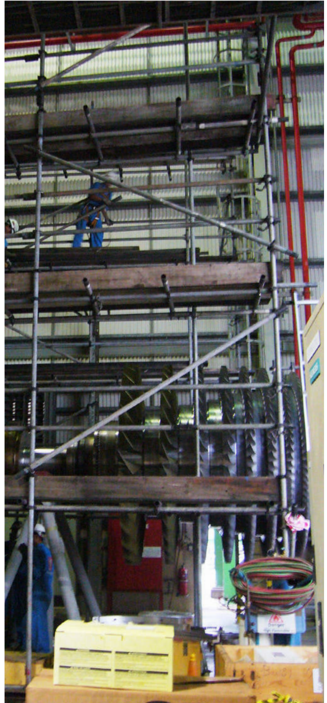
■ BS scaffold tower for GT 94.3 (indoor)
