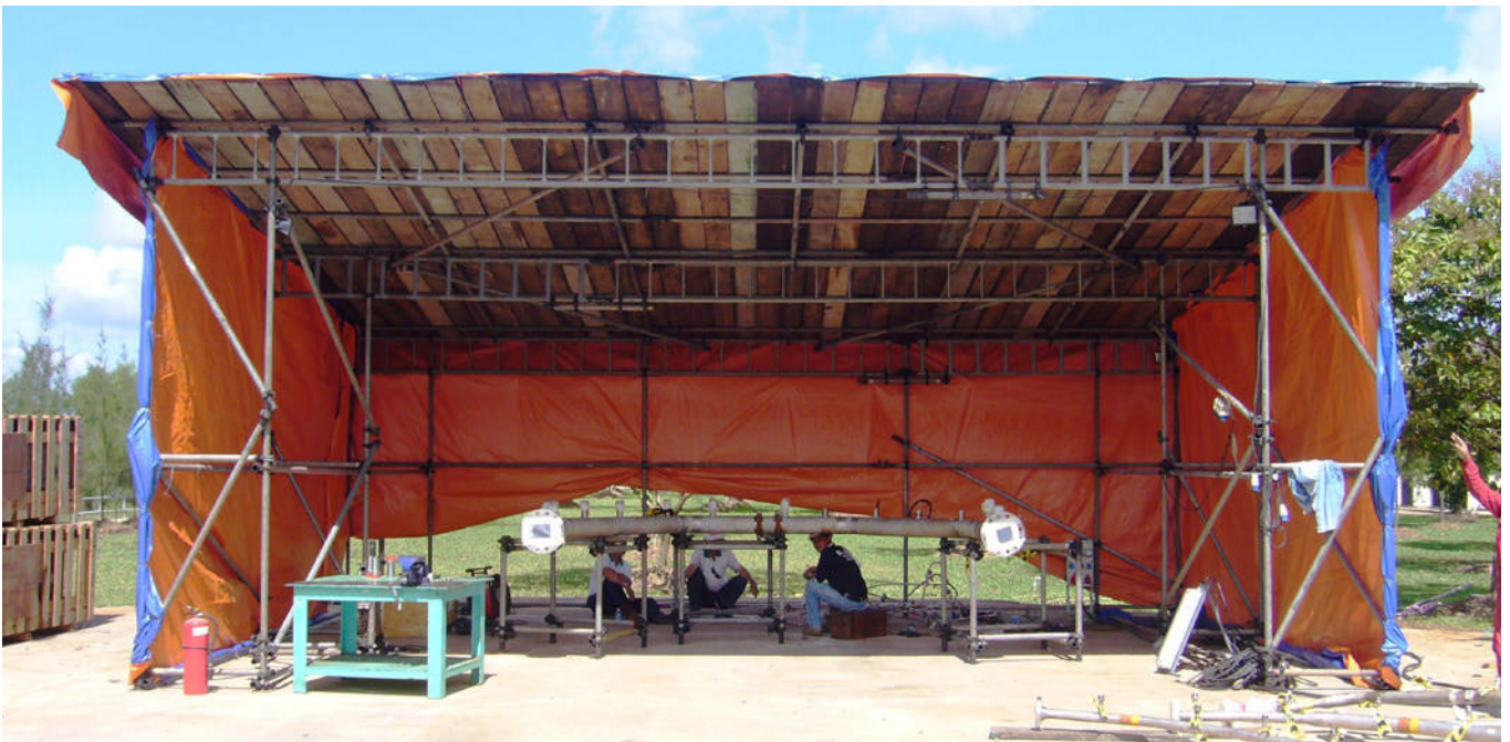
■ Scaffolding shelter for welding works
