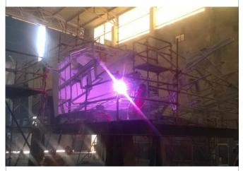
At client's yard, OSV radar mast and deck area have been metallized using both Arc & Flame spray methods following NORSOK standard M-501 requirements.
