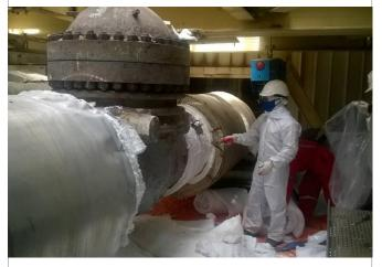
Vivablast has delivered with safety, quality & punctuality BS 1139 scaffolding and insulation remedial works including inspection, removal & replacement on Gas and Steam turbines' lines as well as equipment as part of a Combined Cycle Power Plant shutdown in South of Vietnam.
