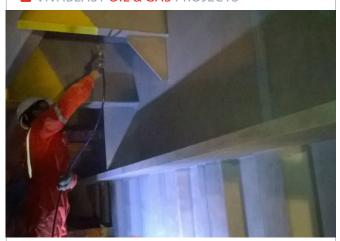
Vivablast has been awarded epoxy intumescent fireproofing system application works for wellhead platform which belongs to the largest petroleum corporation between Russia and Vietnam.
