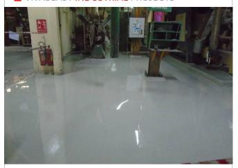
Vivablast has provided heavy duty floor coating services to a major animal nutrition feed manufacturer from floor decontamination with CO2 dry ice cleaning followed by surface preparation and coating to deliver chemical & abrasive resistant flooring system.
