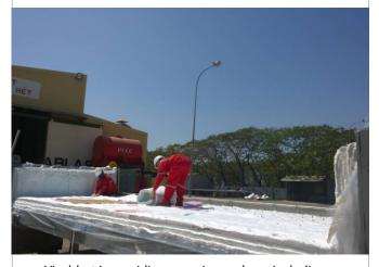
Vivablast is providing a service package including surface treatment, anti-corrosion coating, and internal insulation for power plants dampers. These structures are engineered by a leading international company who had supplied over 10,000 dampers all around the world.
