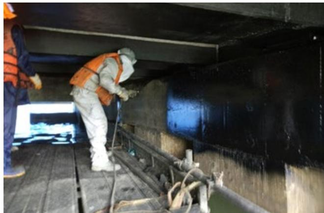
■ **Vivablast** with its expertise in coating application and solution for Jetty protection, has completed another challengeable project at Phu My Port. Since the water level rises while working and allow us for a partial day production; VB has chosen a special product designed for immediate exposure to water and curing under water.
