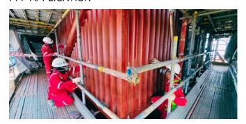
VIVABLAST is honored to perform PFP (Passive Fire Protection) application to protect drilling platforms in Southeast Vietnam. We brought our expertise in Passive Fire Protection to offer the most advanced painting system from recognized intumescent paint manufacturers. In the highly flammable environment of drilling platforms, we made sure to help the client meet the toughest fire safety rules.
