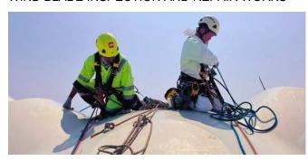
This month, we performed comprehensive inspections of wind turbine blades at nearshore wind farms in Vietnam, including both the interior and exterior surfaces. Utilizing high-quality borescope cameras with high resolution and visual inspection techniques, we conducted a thorough assessment of the blades' condition. Following a repair plan recommended by the client's blade expert, our certified technicians utilized rope access techniques to repair the damages on the blade.
