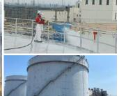
With a proven track record in power generation, VIVABLAST recently executed innovative anti-corrosion coating by employing competent access solutions at a major thermal power plant. Our team of multi-skilled technicians swiftly switched between rope access and scaffolding techniques to effectively access difficult-to-reach areas, such as pipe racks, boiler castings, oil storage tanks, and other structures, enabling them to plan, execute tasks efficiently with the utmost safety and on schedule.
